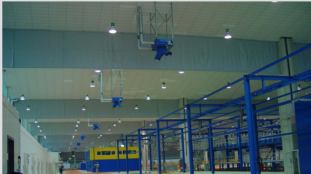
Smokemaster SM-ST smoke curtains are easy to install to the existing structure of the building.
